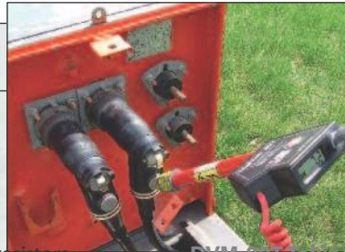
DVM-80T Taking Elbow Test Point Measurement
